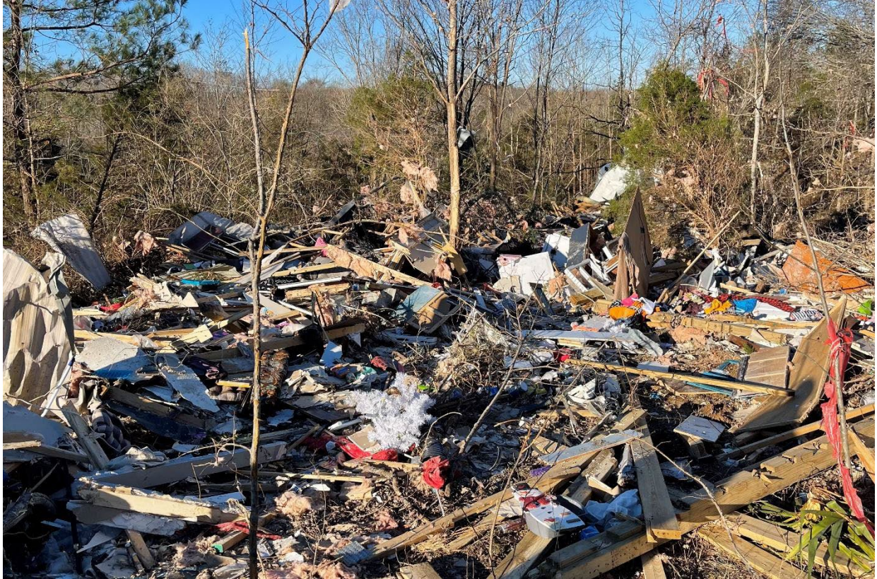
Figure 22: Stewart County tornado damage (Source: Stewart County EMA)
